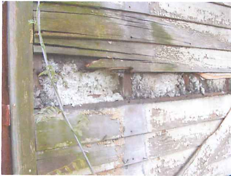
Photo M2 Structure #2234 - Typical Wall Framing of Building #2234
