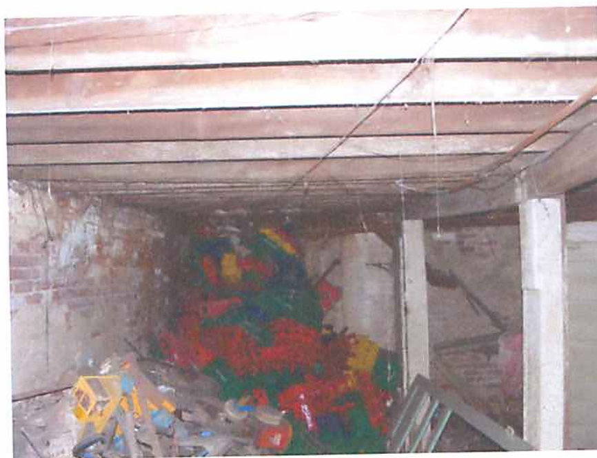
Photo R10 Structure #2238 - Post, Beam, Joist First Floor Framing
