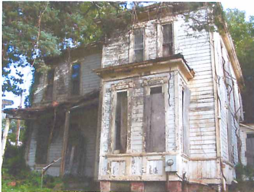
Photo L12 Structure #2228 - Front of Building #2228
