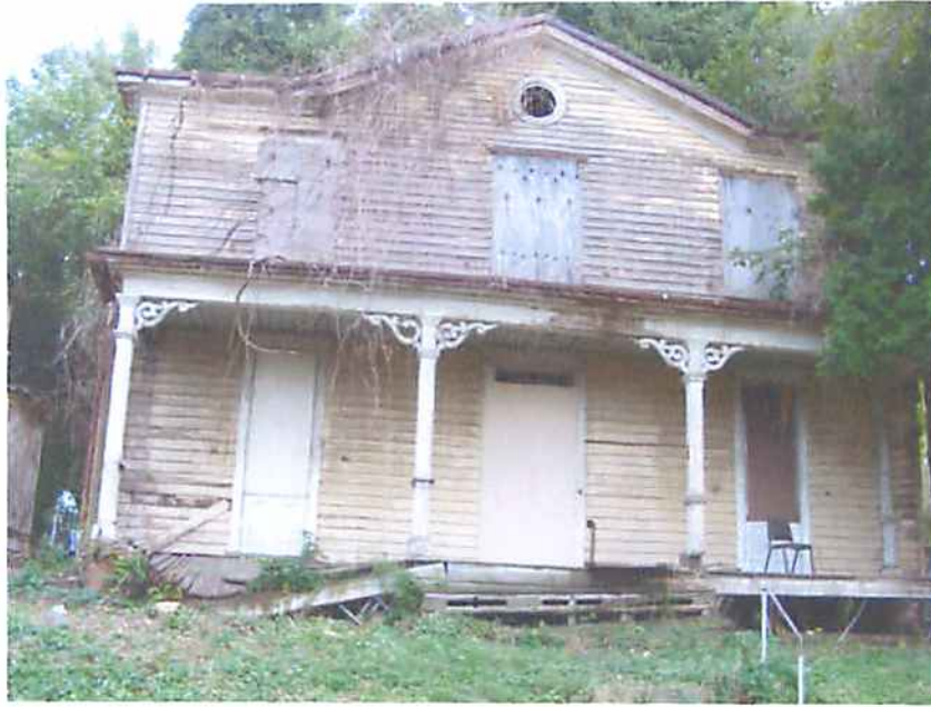
Photo M1 Structure #2234 - Front of Building #2234
