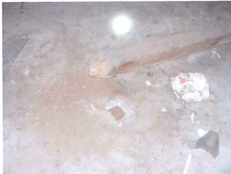
Photo R12 Structure #2238 - Collapsed Post Between Basement and First Floor Framing - Base of Post Deteriorated - Typical Condition For All Basement Wood Posts
