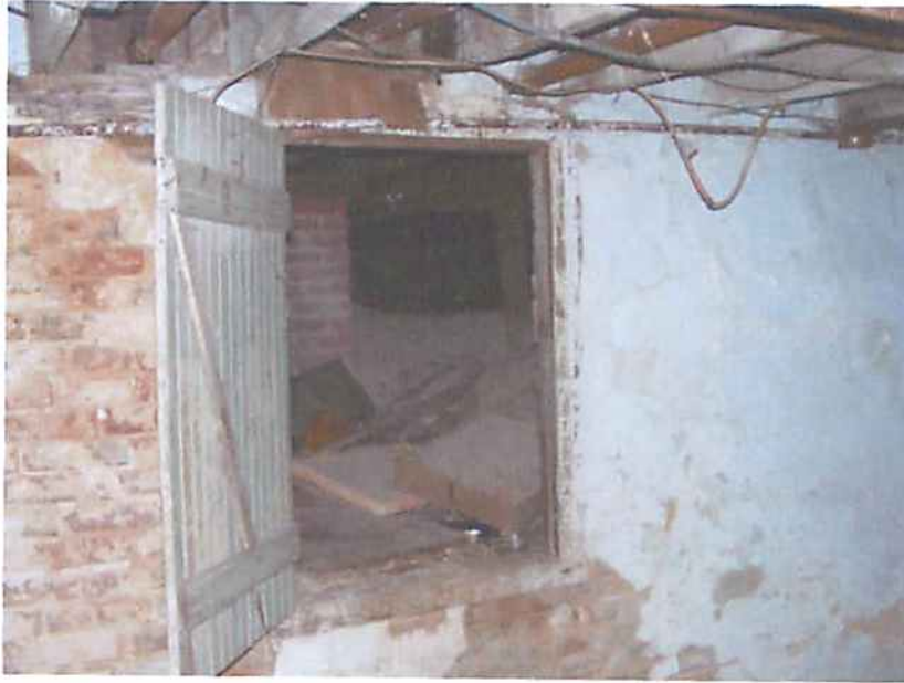
Photo L1 Structure #2228 - Access Opening to Crawl Space
