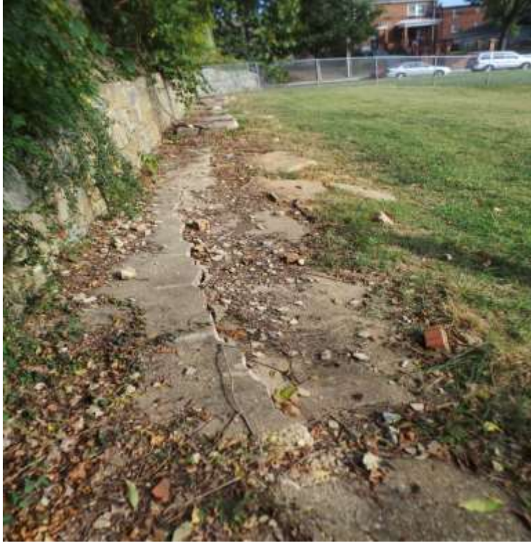
Concrete slabs along the West side of the Site
