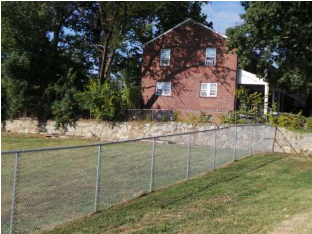
Stone-wall on the West side
