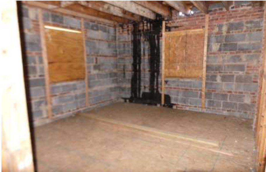
Roof Tar on Wall in Residential Unit on Second Floor
