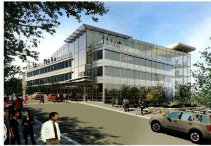
SHANNON PLACE OFFICE BUILDING
