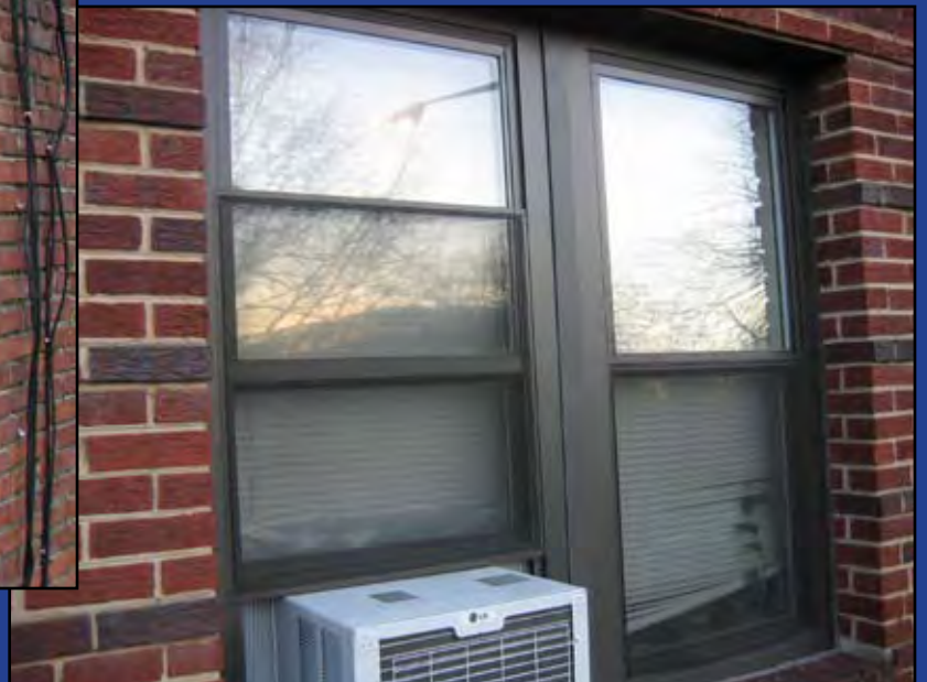
841 19th Street Window Detail Post-Renovation
