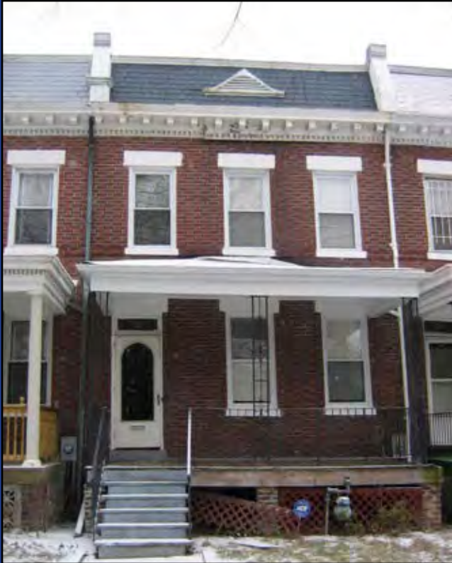
Front View Post-Renovation
