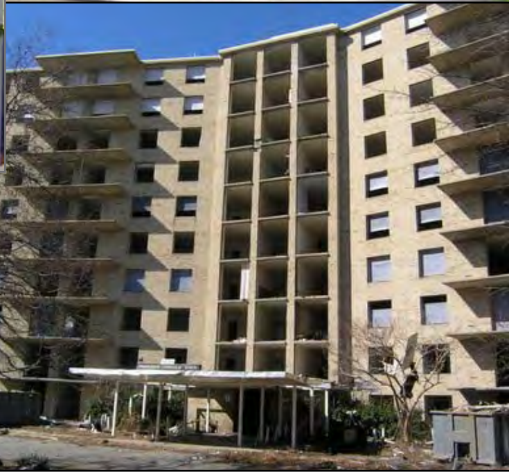
Parkside Terrace/The Overlook at Oxon Run Pre-Construction
