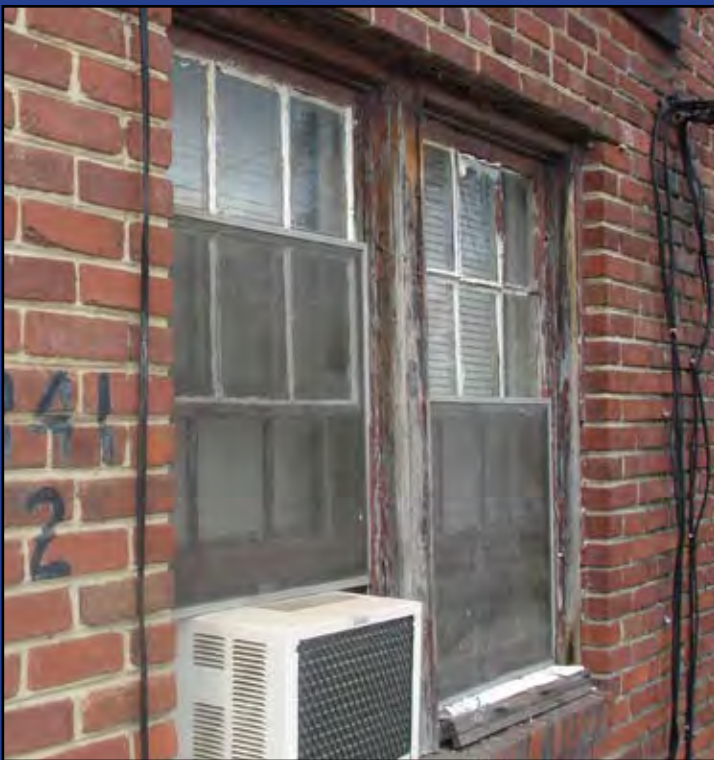
841 19th Street Window Detail Pre-Renovation
