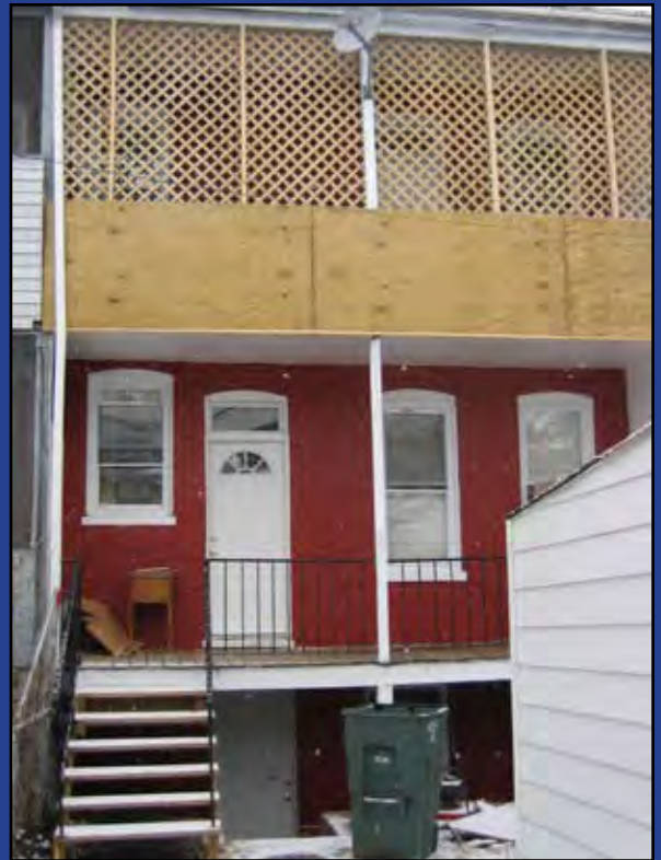
Rear View Post-Renovation
