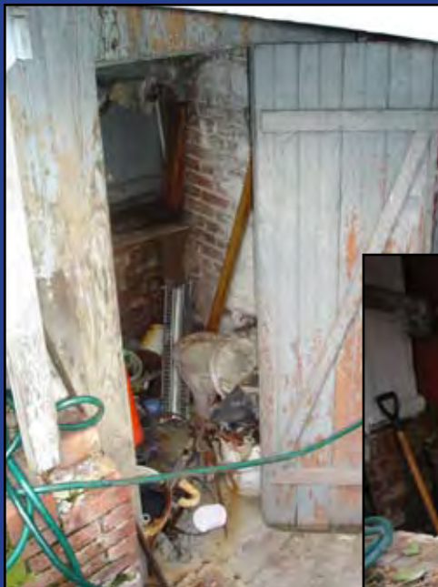
Under Rear Porch Pre-Renovation
